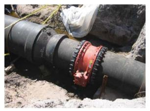
**4.4 New Valves in Existing Mains:** Special cutting-in valves and sleeves are commonly used by water utilities and contractors to install
