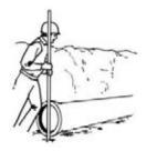
4. Small pipe can be pushed into the bell socket with a long bar. Large pipe requires additional power, such as a jack, lever puller, or backhoe. The supplier may provide a jack or lever puller on a rental basis. A timber header should be used between the pipe and the jack or backhoe bucket to avoid damage to the pipe.
