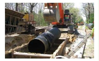
**1.4 Slings:** A variety of slings are available for handling pipe. Nylon slings, with an appropriate lifting capacity, are particularly well-suited for lifting Ductile Iron Pipe and appurtenances.
