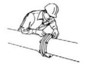
3. Push the gland toward the socket and center it around the plain end with the gland lip against the gasket. Insert bolts and hand tighten nuts. Make deflection after joint assembly but before tightening bolts.
